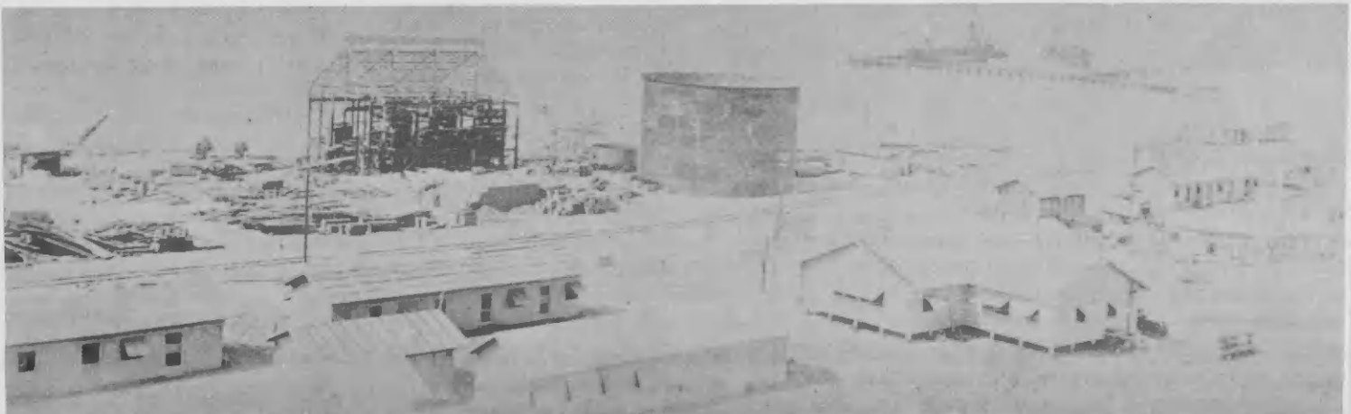
The tank shown here is probably the first built at Lago.
